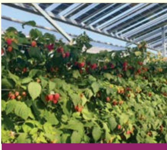
Pictured: Agricultural Photovoltaics fixed shade system over raspberry farming.
